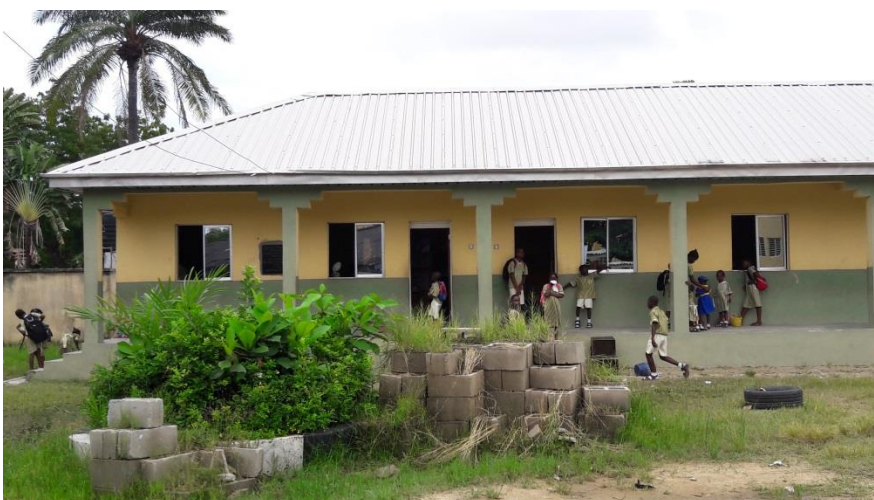
A typical classroom block
