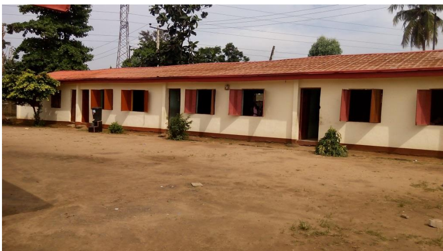
A typical Classroom block in Ilupeju Public Primary School
