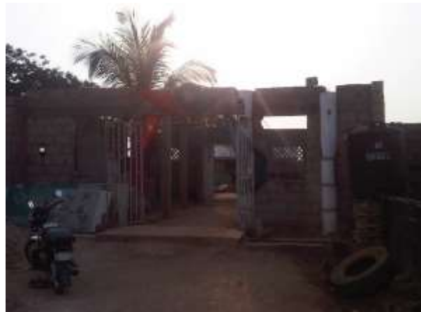
Other facilities under construction
