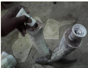
Fig(L):Installation of Lamp Holder
