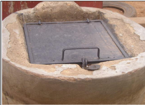
Fig. 6: Ringed and covered well at Ikare
