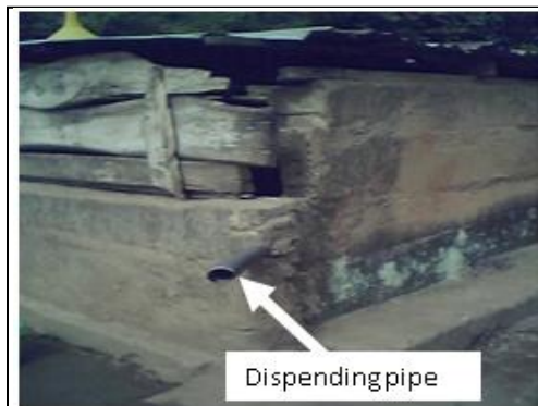
Fig. 11: Pond protection with concrete walls, planks and iron sheets at Ikare
