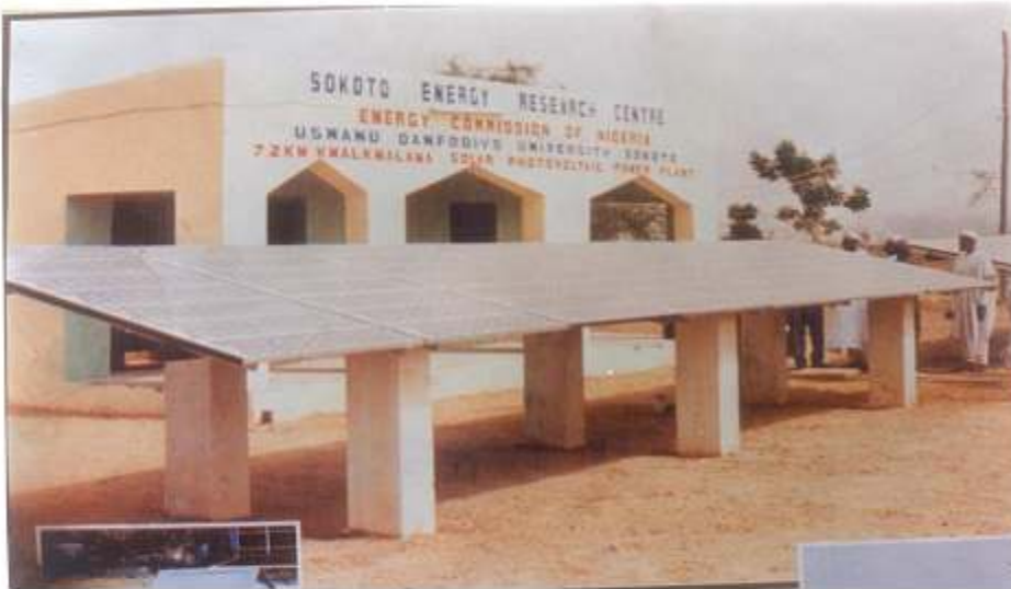
7.2 kWp PV Village Electrification, Kwalkwalawa, Sokoto State by SERC
