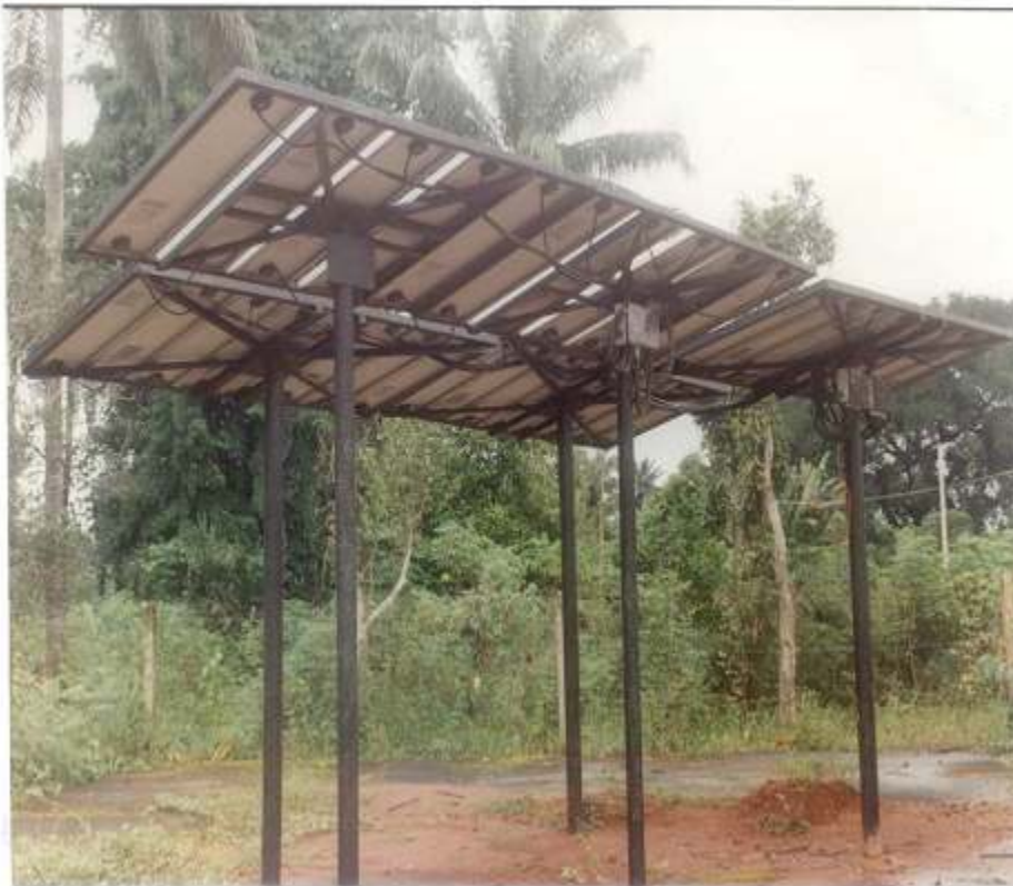
Figure. 14: 1.87 kWp PV Village Electrification & TV-Viewing Plant Iheakpu-Awka, Enugu State by NCERI
