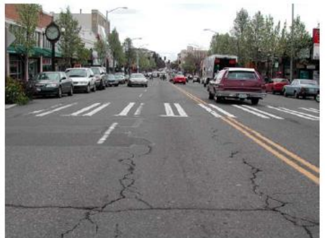
Plate 6: Pavement in Fair Condition Cracking is extensive and the pavement surface is weathered. The pavement shows signs of structural damage.
