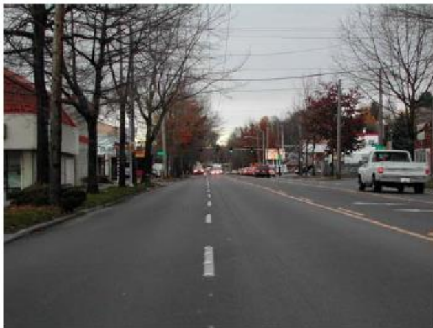
Plate 5: Pavement in Excellent Condition The pavement is smooth and generally free of distress.
