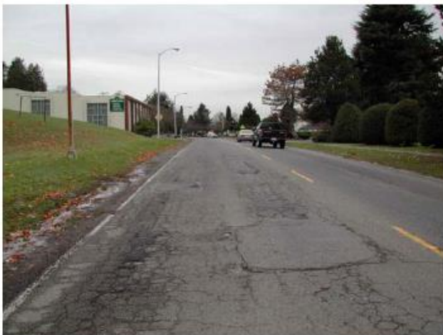
Plate 7: Pavement in Very Poor Condition The pavement surface is cracked and disintegrated. Structural damage is widespread. The ride has deteriorated to the point where traffic operations are affected.
