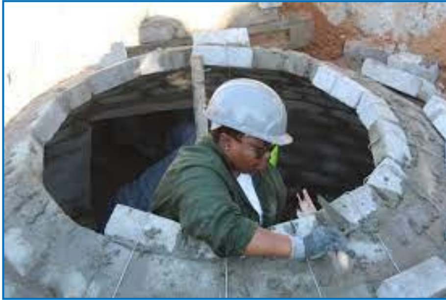
Plate 2: Construction of biogas digester Source: UNDP, 2020
